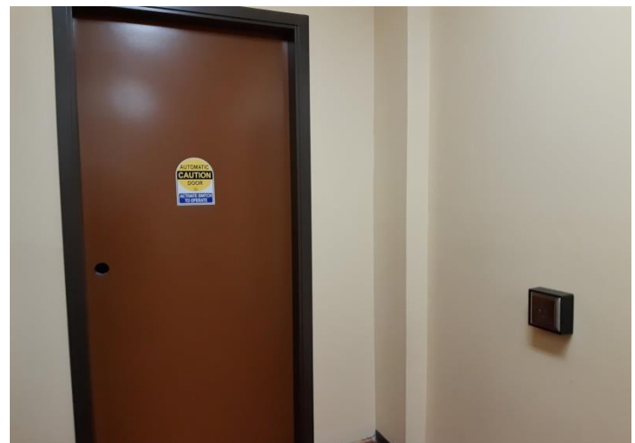
Automatic door is in place and operational
